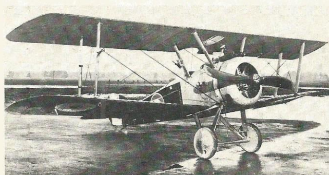
Below: Probably the most famous aircraft of W.W.I, the Camel (F.1 version illustrated) is the type credited with destroying the greatest number of enemy aircraft—1,294. It will also be remembered for the rapidity of its right-hand turns—due to the gyroscopic force of its rotary engine. Production totalled 5,497 (Photo: Imperial War Museum)
